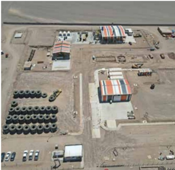
↑ Kal Tire's tyre recycling facility in Chile
